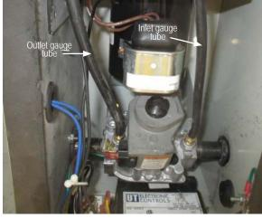
Single stage valve shown for representation of gauge tubing connection.
