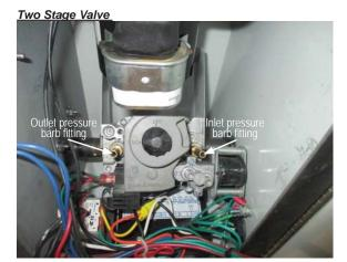
3. Route gauge tubing through burner box air inlet to gas control valve. See Fig. 17.
