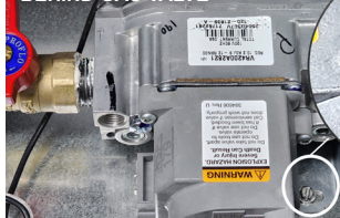
2ND SCREW BEHIND GAS VALVE
