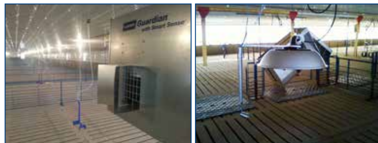
Works with a wide range of house controls that offer a 0-10 volt signal.
