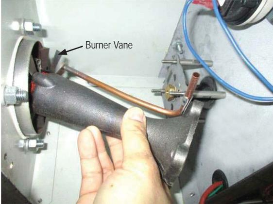
4. Remove orifice and burner inlet plate See Fig. 4.
